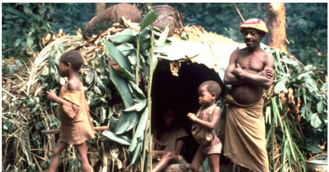
The hemispheric hut of the Baka is exclusively made of vegetal materials and is built by women in just a few hours. This ephemeral construction offers protection against night cold and mosquitoes (Photo by Edmond Dounias)
