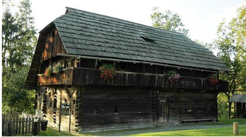
Figure 5: The „Bodnerhaus“ is the oldest blockhouse in Austria, Carinthia built around 1470, located in the Freilichtmuseum Maria Saal with a typical dark wood-patina due to ageing (@kultur.net)
