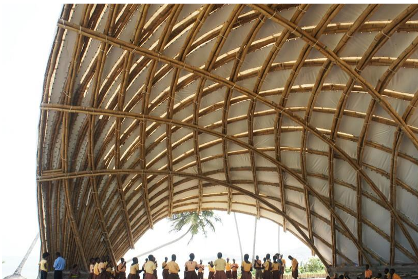
Figure 18: Haduwa arts + culture institute in Ghana protected by dynamic bamboo canopy (Source: https://www.designboom.com/ )
