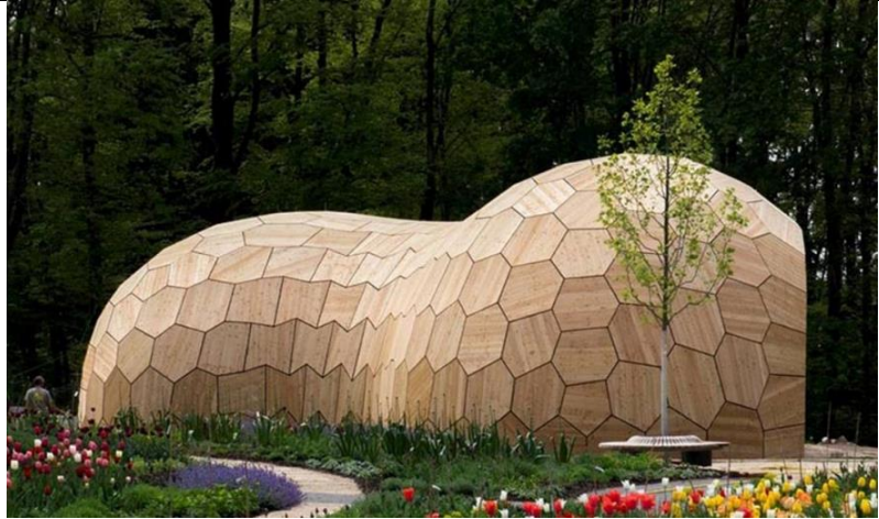
Figure 4: Peanut-shaped exhibition hall Landesgartenschau Schwäbisch-Gmünd, Stuttgart, Germany (robotic fabrication) by University of Stuttgart (@Institute of Computational Design's (ICD))
