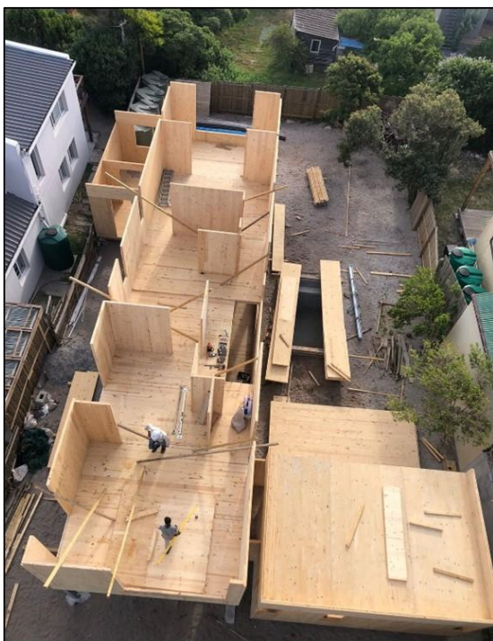
Figure 16: Example of CLT-based construction in South Africa (Source: TheWoodApp, 2023; Pinto, 2021)
