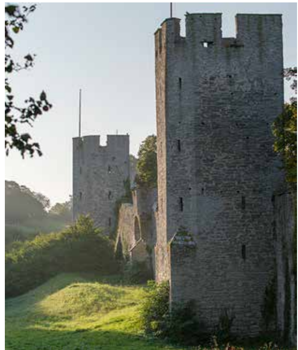
A medieval defensive city wall surrounds the town of Visby, Gotland. Photo: Emelie Asplund/imagebank.sweden.se.
