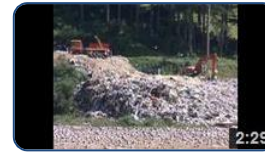
TERAX pilot plant
