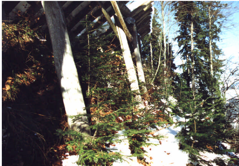
Figure 1: Snow rakes protect young firs against snow movements
