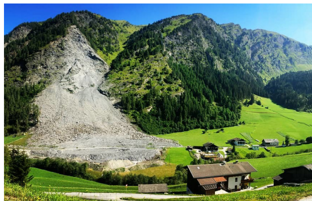
Rock avalanche in the GreenRisk4ALPs Pilot Action Region “Gries am Brenner / Vals” in Austria, endangering infrastructure, adjacent to protective forest reducing rockfall risk. Photo: Barbara Žabota, University of Ljubljana
