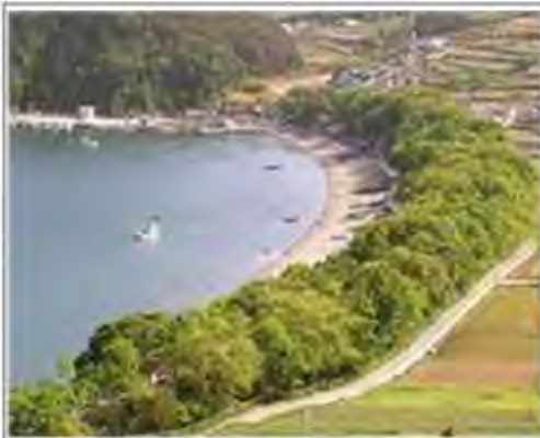
A work to create a forest for damage prevention along the beach
