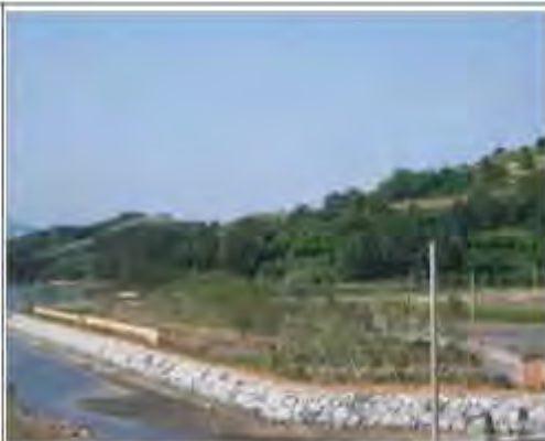
A work to prevent coastal erosion
