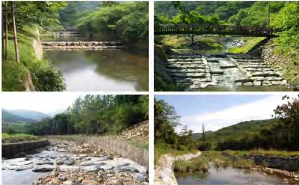
Inter-stream grade stabilization structures, channel, revetment using vegetation sacks, introduction of aquatic organisms around project site
