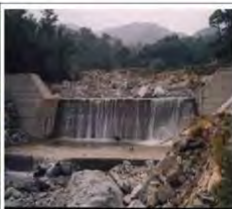
A construction work of an erosion control dam
