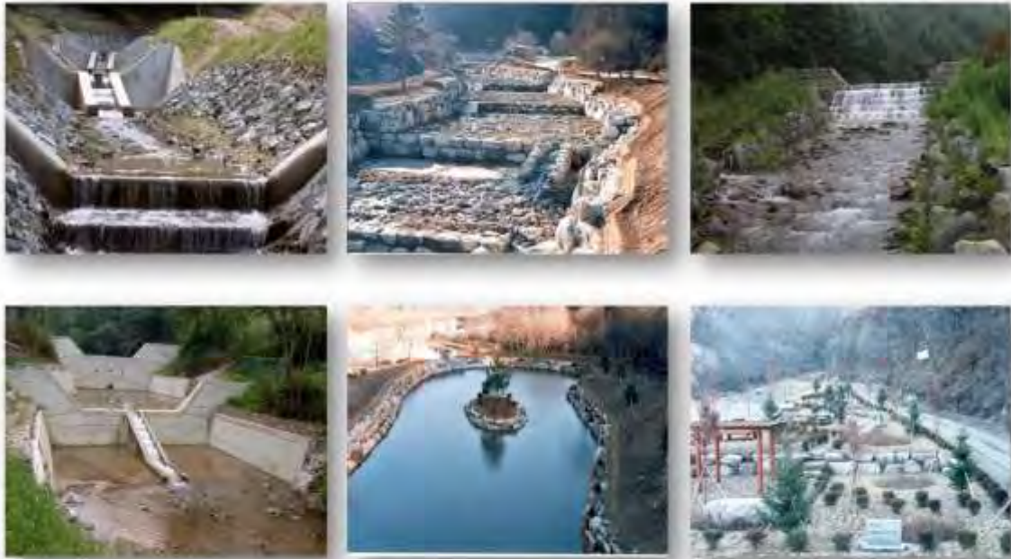
Eco-friendly Erosion Control Works
