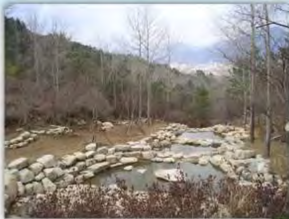
A mountain stream conservation work (Gyeongnam)
