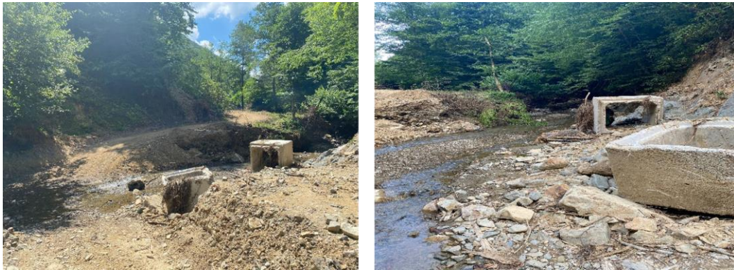
Figure 2. The current status of the box culvert
