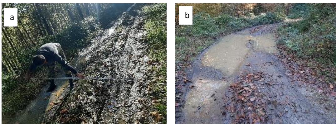
Figure 4. Uncontrolled recreational use led to severe erosion on road surface
