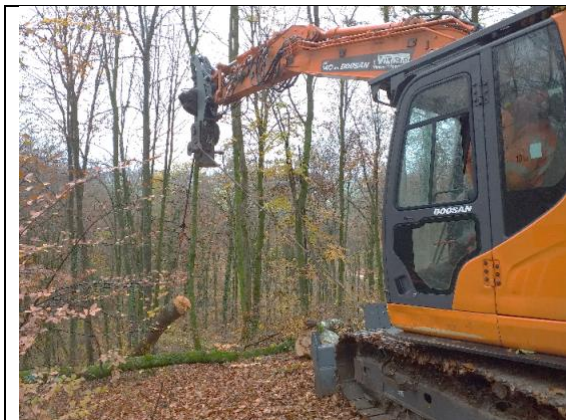
Figure 5 : Hub here in vertical position while using the cable-lifting pulley
