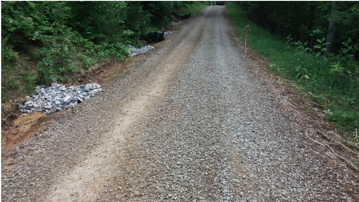
Figure 1. Two experimental units at one cross drain, separated by silt fence. The closest two check dams and silt fence are the second experimental unit. Picture was taken Pre-harvest (June 2014).
