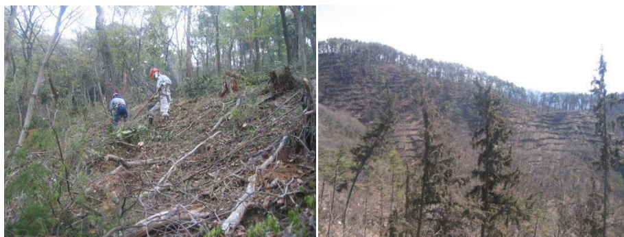
Figure 2. Forested hillside site preparation (left), and terrain after site preparation (right).
