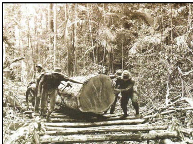
Figure 6. Pulling log using kuda-kuda system in 1963 in peat swamp forest. (Source: Forestry Department Peninsular Malaysia, 2001).
