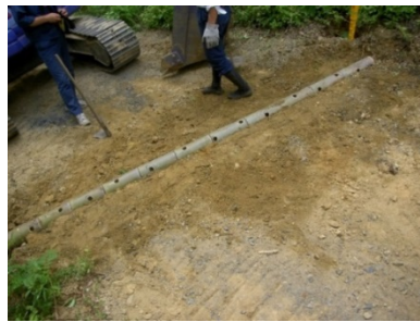
Photo 2: Cross ditch made with a node-free Moso bamboo culm, with drilled holes for water passage
