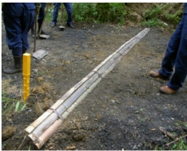
Photo 1: Cross ditch made with stripped Moso bamboo
