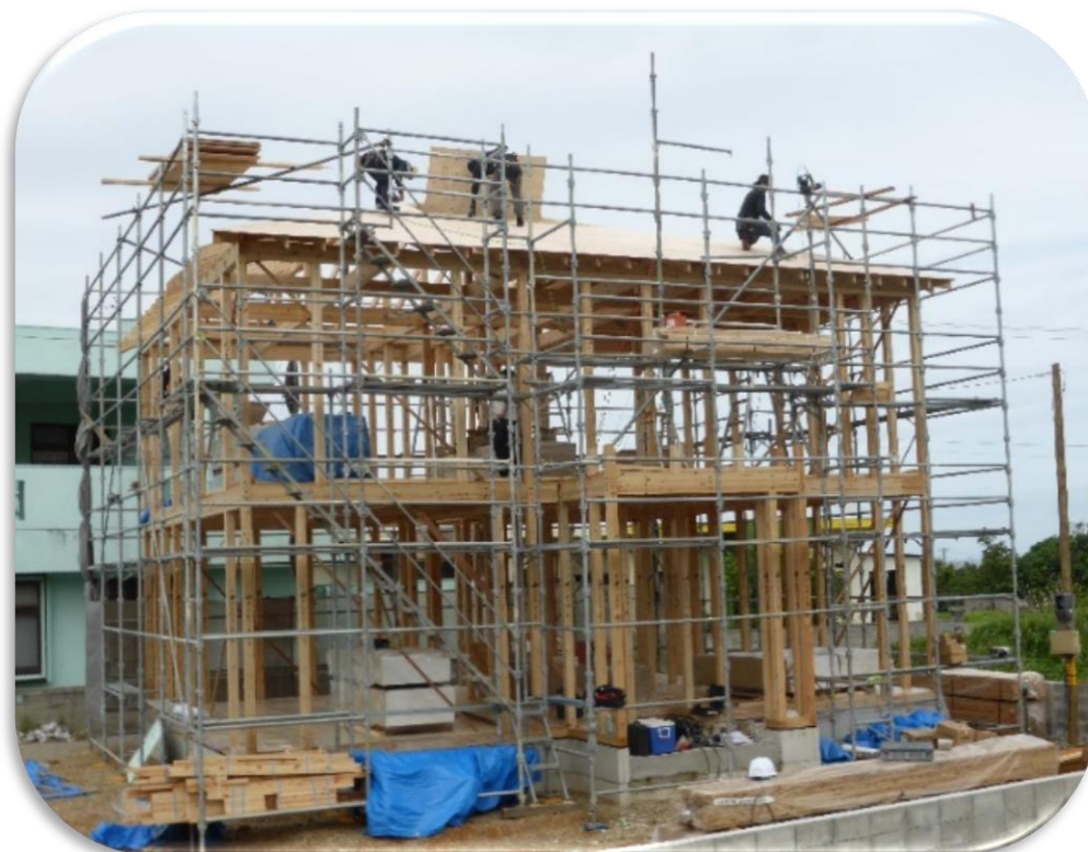
Figure 3. Japanese traditional wooden house
