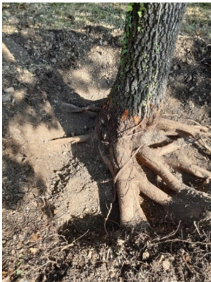
Figure 4 —The exposed root structure of the oak tree before systematically severing each of the main roots
