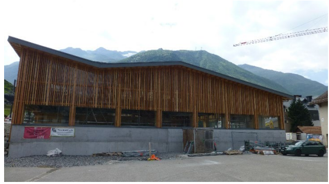
Figure 2 – cable car station in Andermatt, Switzerland at an altitude of 1500 m.a.s.l.
