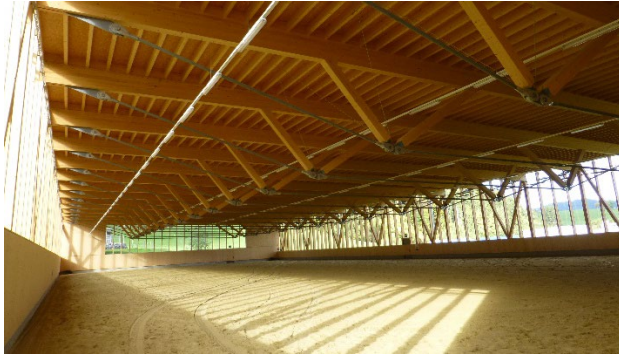
Figure 1 – View on the interior of a riding hall located in Einsiedeln, Switzerland
