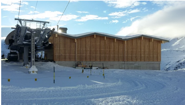
Figure 3 – View on the cable car station of Nätschen, Switzerland at an altitude of 1850 m.a.s.l.
