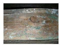
Figure 6: Extensive infestation by *Trichoderma viride* on a beam in the Rococo Hall before restoration
