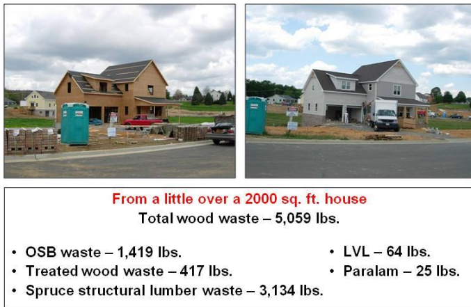
Figure 1 Example of the amount of wood waste generated from new home construction on Lot #47
