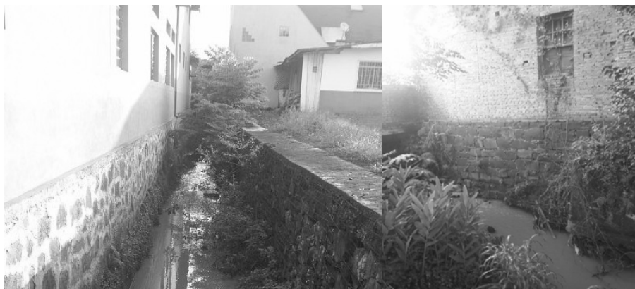
Photo 1 - Margins of Arroio dos Pereiras on May 24 Avenue. Author: Campos, 2006.
