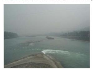
leads the water into the Chengdu Plain. The bed of the outer river is convex while that of the inner river is concave. This fact, an integral part of Li Bing's original design, results in less silt going into the inner river, which is primarily used for irrigation.
