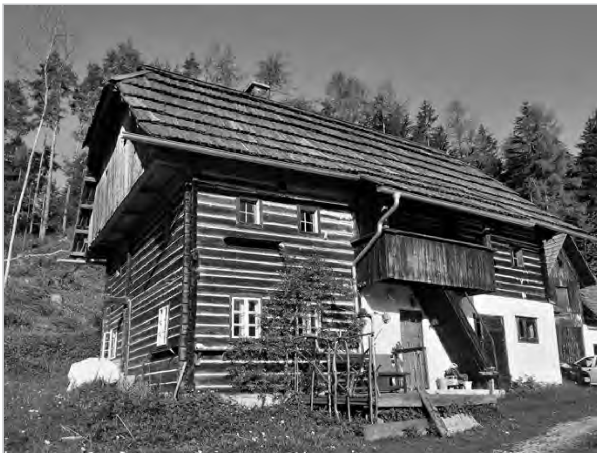
Figure 2: Wooden log-house in the Southern Austrian Alps from the early 18th century. Beside the stonewall-stable the building material is larch, harvested in the close surroundings. The house was part of a hammermill and is inhabited till present day (Photo E. Johann)
