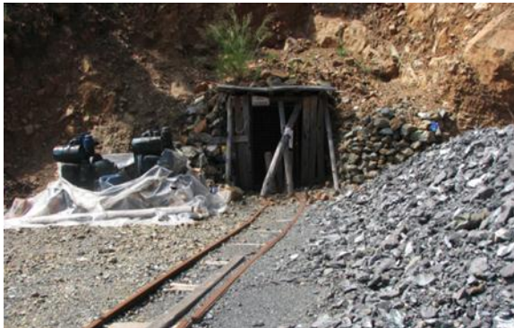
Picture 4. Mining gallery entrance 1
