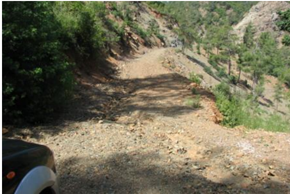
Picture 2. Forest Road to Mine site
