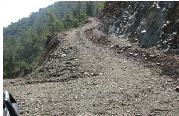
Picture 3. Forest Road to Mine site
