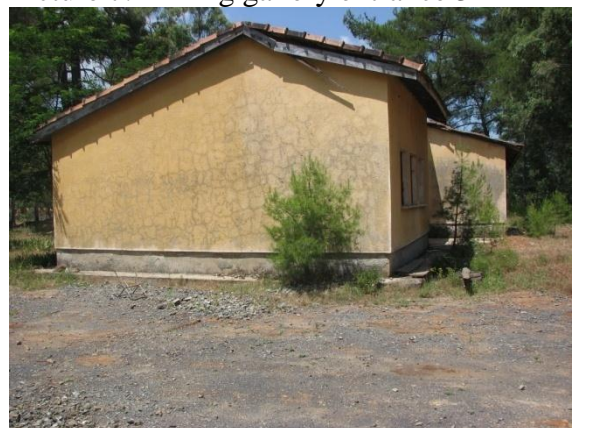
Picture 9. Administration building (Outside the Wildlife area)
