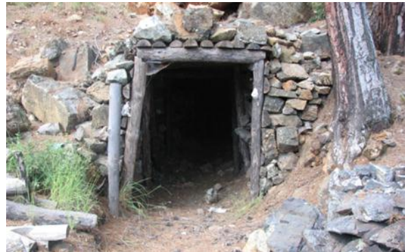
Picture 5. Mining gallery entrance 2
