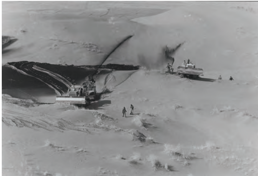
Figure 12: Using mulch for fixation of sand dunes in Iranian deserts (Photo taken by Darvish)
