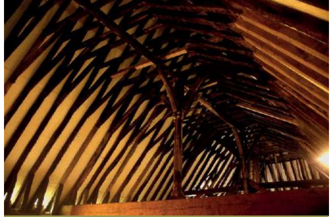
Photograph 35: A roof probably of the 14 th century CE. Each timber represents one small oak-tree. Medieval woods were managed for a continuous supply of such trees (Canterbury, England).
