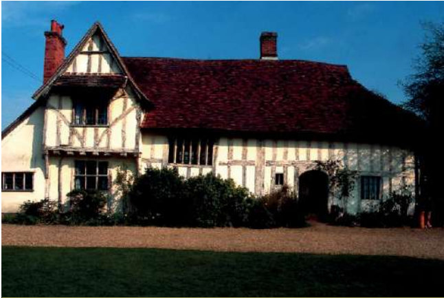
Photograph 36: An ordinary timber-framed house of c. 1400 CE. The timber frame is made partly of cheaper species than oak, and of recycled timbers. The spaces between the timbers are filled with coppice poles covered with clay (Flatford, Suffolk, England).
