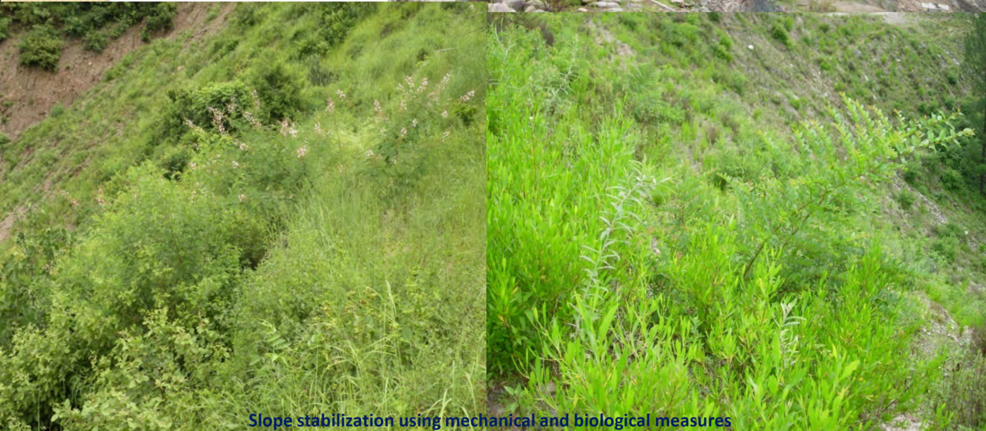
Slope stabilization using Mechanical measures
